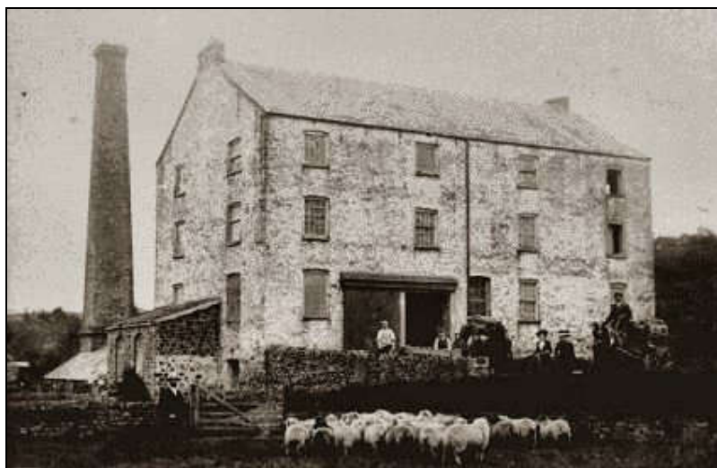
The former Lower Woollen Mill c 1900 – converted to flats c 1990s
